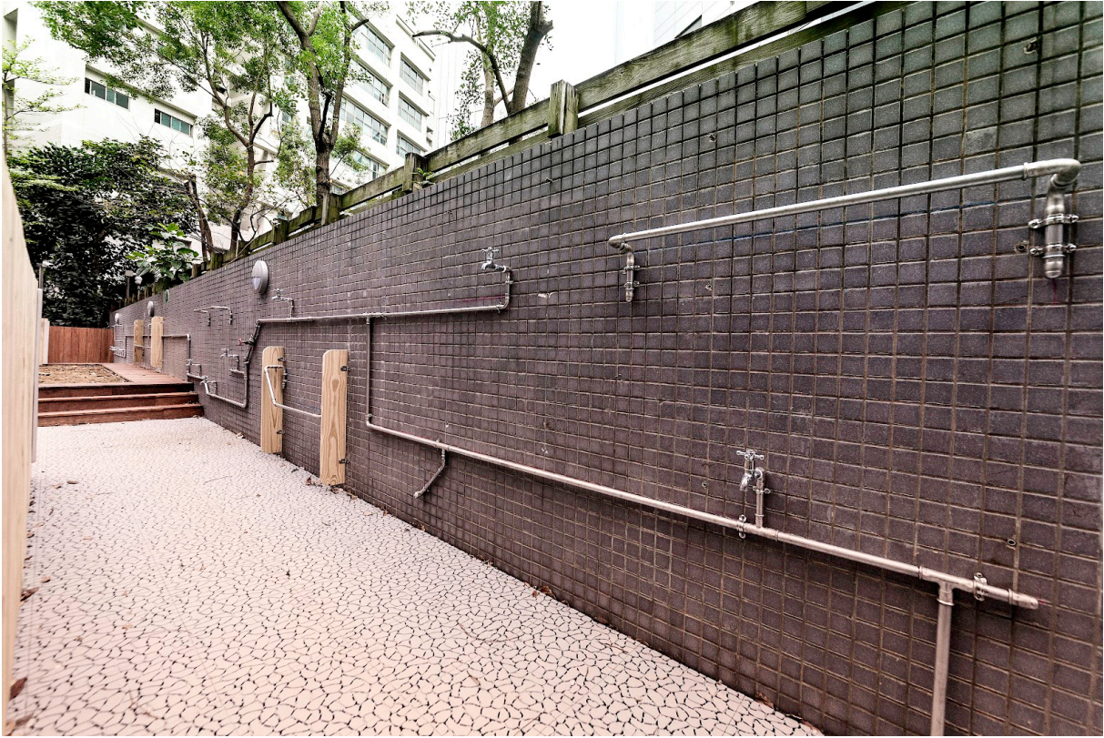
▲The outdoor sandpit combines the faucet installation art, which is both practical and beautiful.
